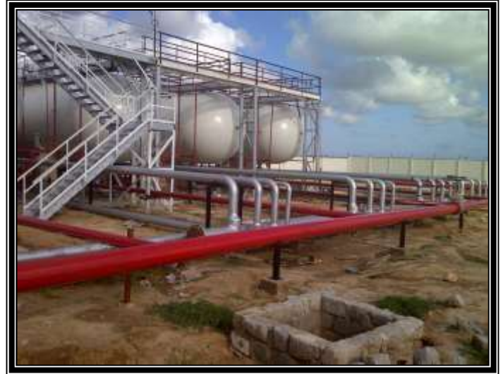
AGOL LPG PIPE CONSTRUCTION KENYA
