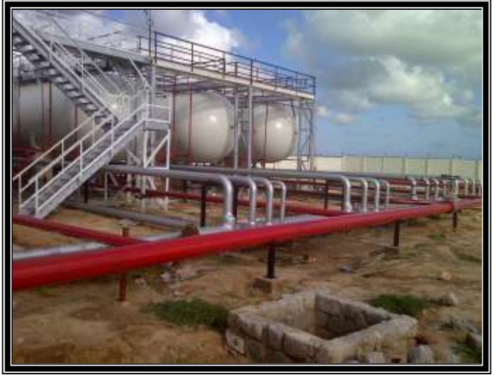
AGOL LPG PIPE CONSTRUCTION KENYA
